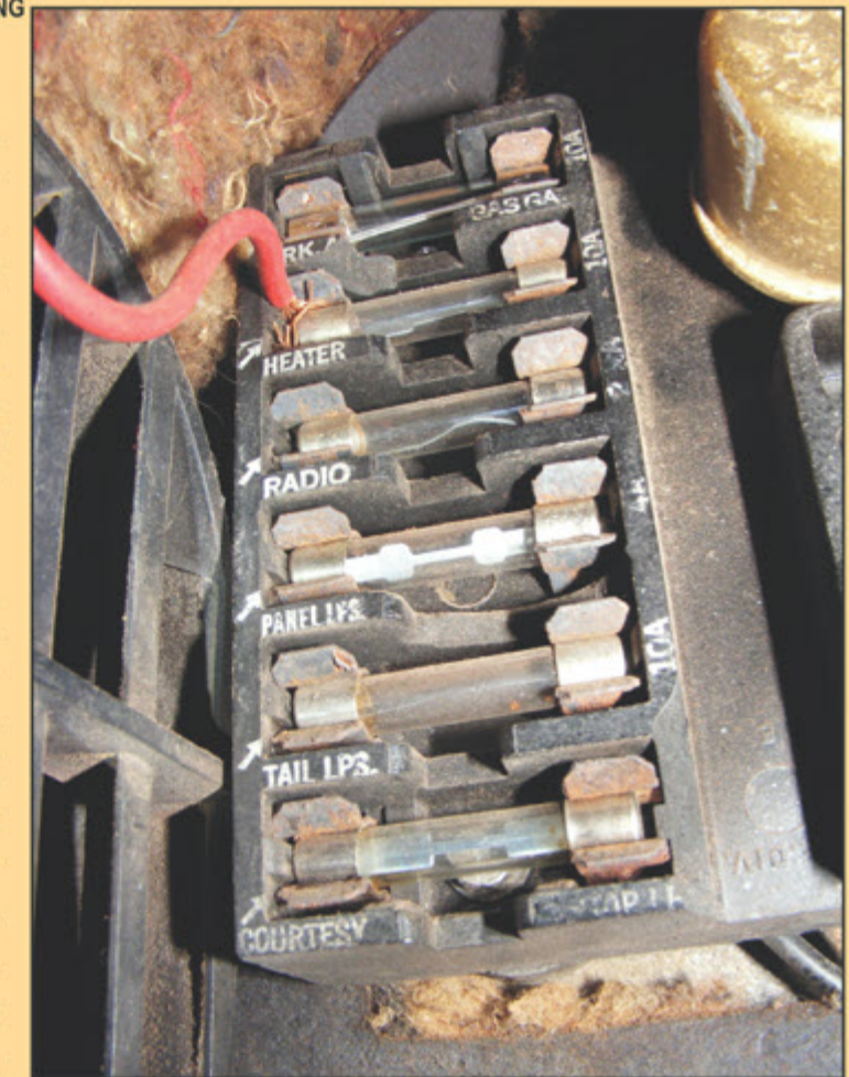
1964 CORVETTE FUSE BOX
