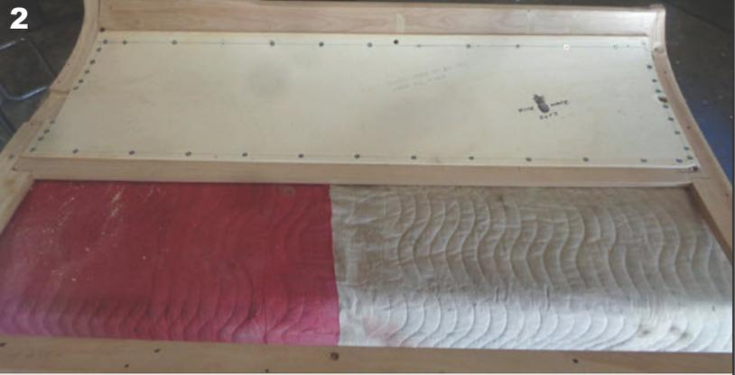
fit I marked a 1/2 inch margin all the way around the wood insert and made sure I was good on the door frame with a good margin on it. •I centered the screws and marked off every 4
